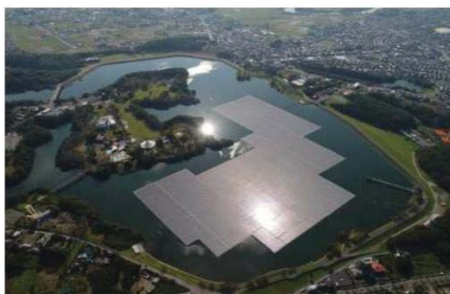
Fig. 5 Yamakura Dam Reservoir FPV System (13.7MWp) [17]
