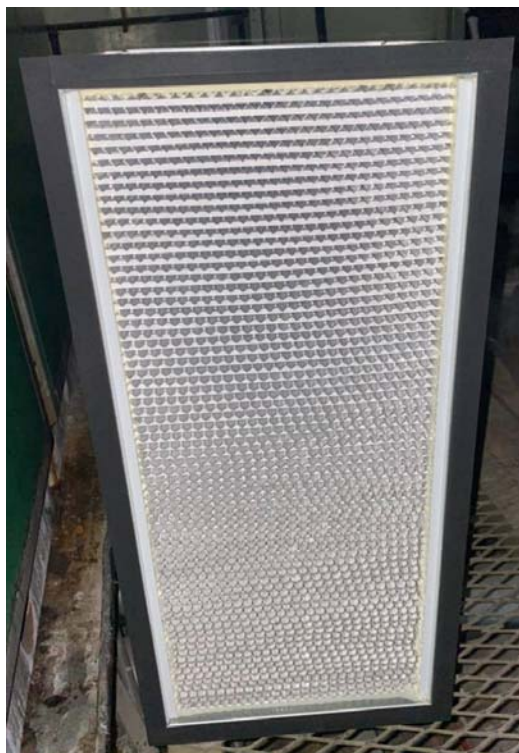
Fig. 10 HEPA filter
