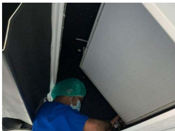
Fig. 11 HEPA unit installation
