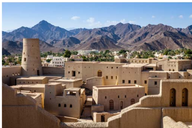
Fig. 1 Some features of the vernacular Omani architecture; solidity, simplicity, small screened windows, grouped and joint units [25]
