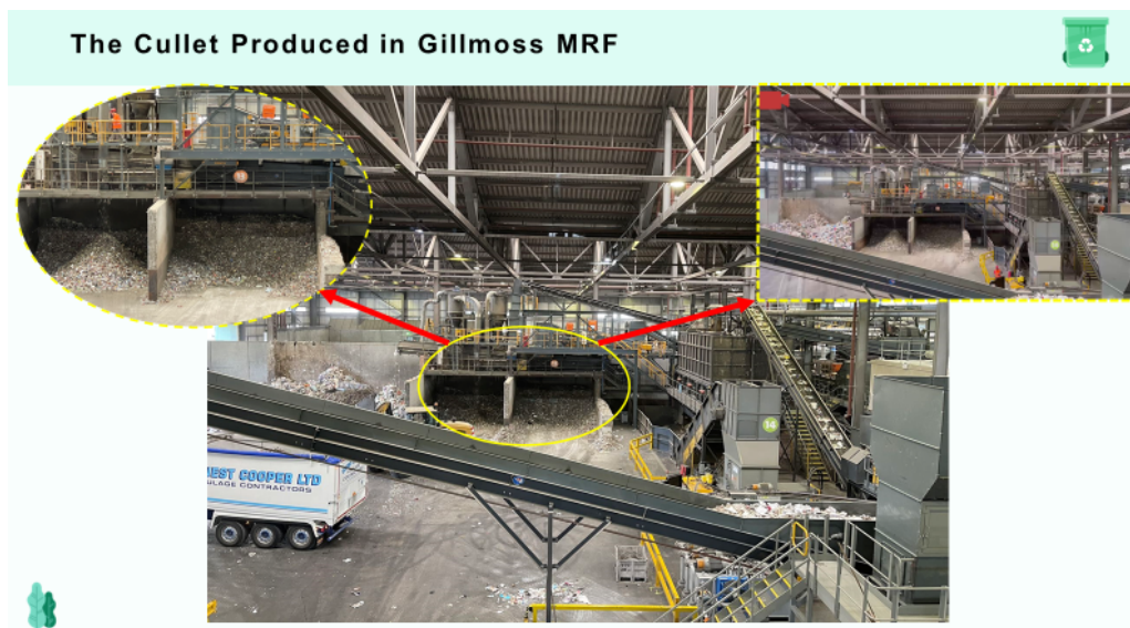
Fig. 6 Step 3) Cullet produced after glass breaking process in Gillmoss MRF
