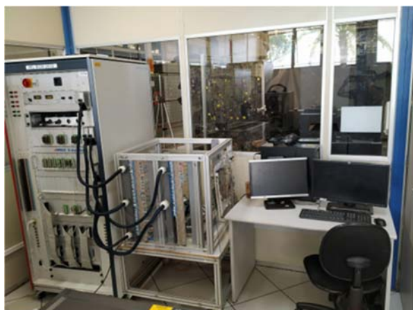
Fig. 13 ECU and Simulator Connection in Platform
