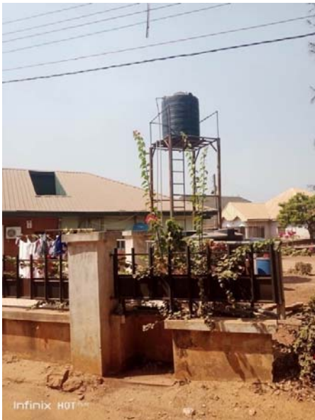
Fig. 2 A household using an overhead water tank connected to a borehole due to non-access to the central water supply
