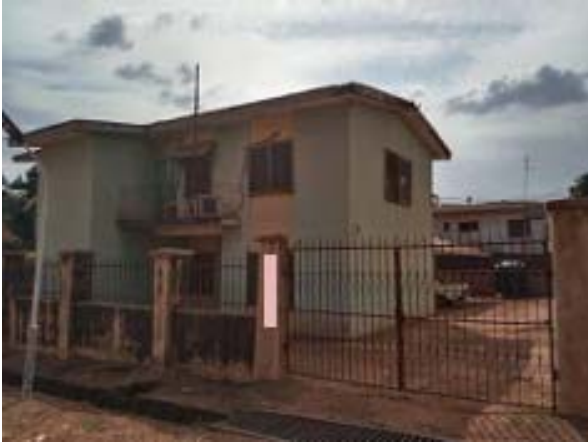
Fig. 1 A residential housing in the Abakpa housing property in Enugu with decaying roof, windows and weakening fence walls
