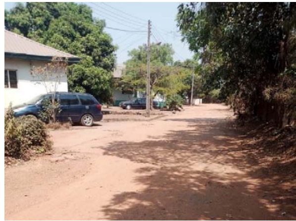
Fig. 3 A street in a government housing property in Enugu with unpaved access road and no drainage channels
