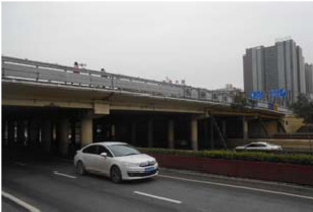
Fig. 1 Outside view of Chang'an Road Interchange
