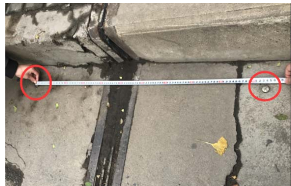
Fig. 6 Measuring point of expansion joint width
