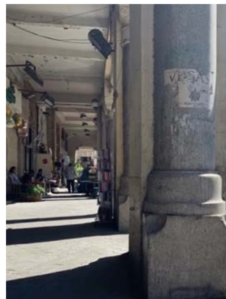
Fig. 16 Baghdad Street arcade, 2021 (taken by author)
