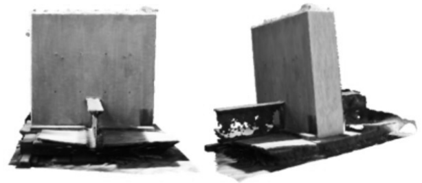
Fig. 10 (b) Northern and North-Western view of wall
