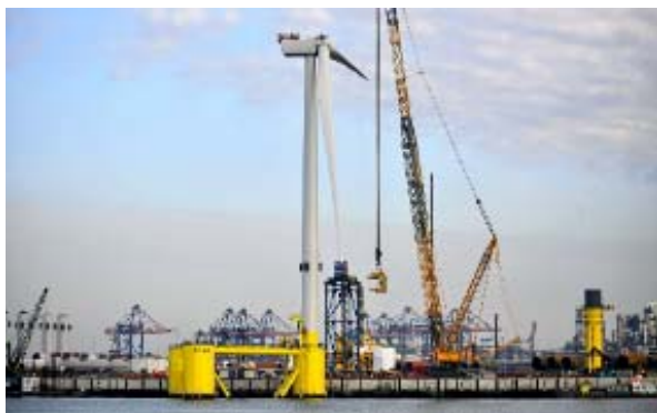
Fig. 10 Blade lifting [13]
