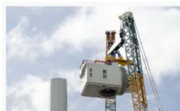
Fig. 9 Nacelle lifting [5]
