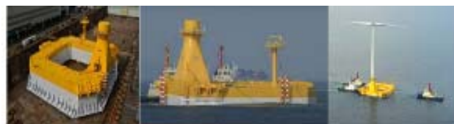
Fig. 13 Steel (damping) barge construction
