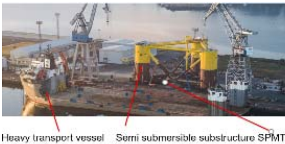
Fig. 3 Semi sub. loadout from land [12]
