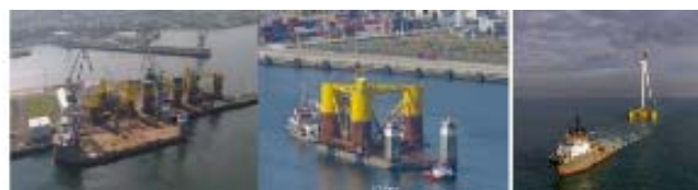
Fig. 12 Steel semi submersible construction
