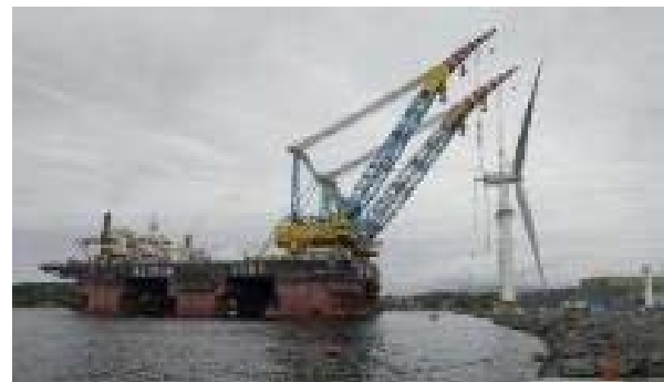
Fig. 6 Spar topsides lift off quay
