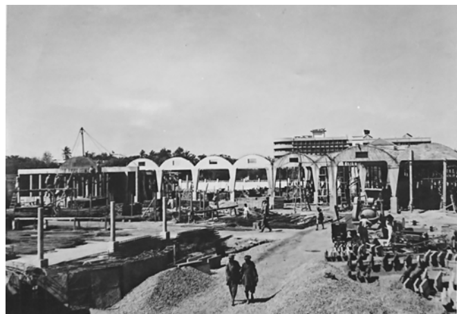
Fig. 4 Construction of the US Embassy in Karachi. c. 1959. Photo: Lucien Herve [29]
