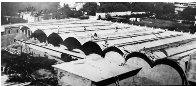
Fig. 8 U.S. Embassy in Karachi under construction, c. 1959. © Neutra Family [29]
