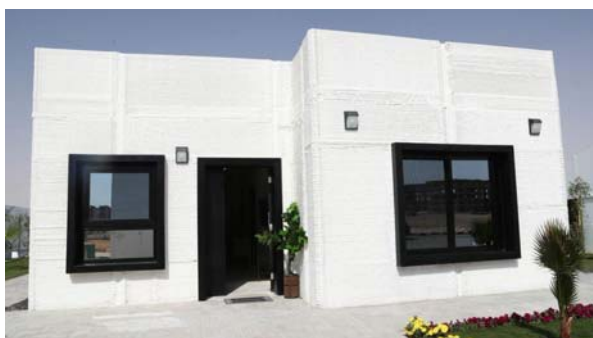
Fig. 4 The first 3-D printed House in KSA by the ministry of housing in collaboration with Cybe [8]
