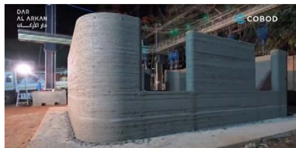
Fig. 5 Dar Al-Arkan 3-D printed structure with COBOD technology
