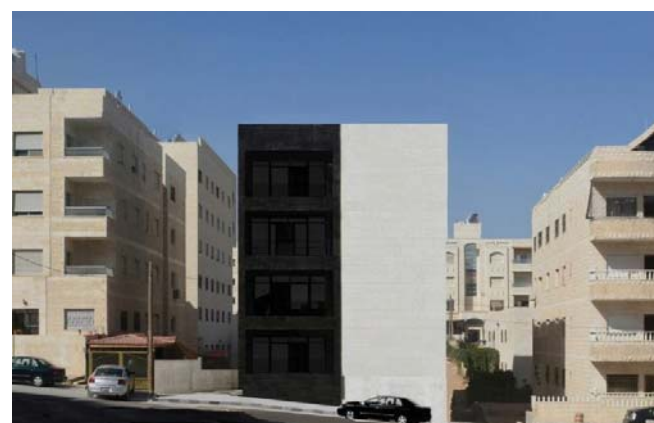
Fig. 8 Ard 334 Apartment Building, 2017, Amman, Jordan [4]
