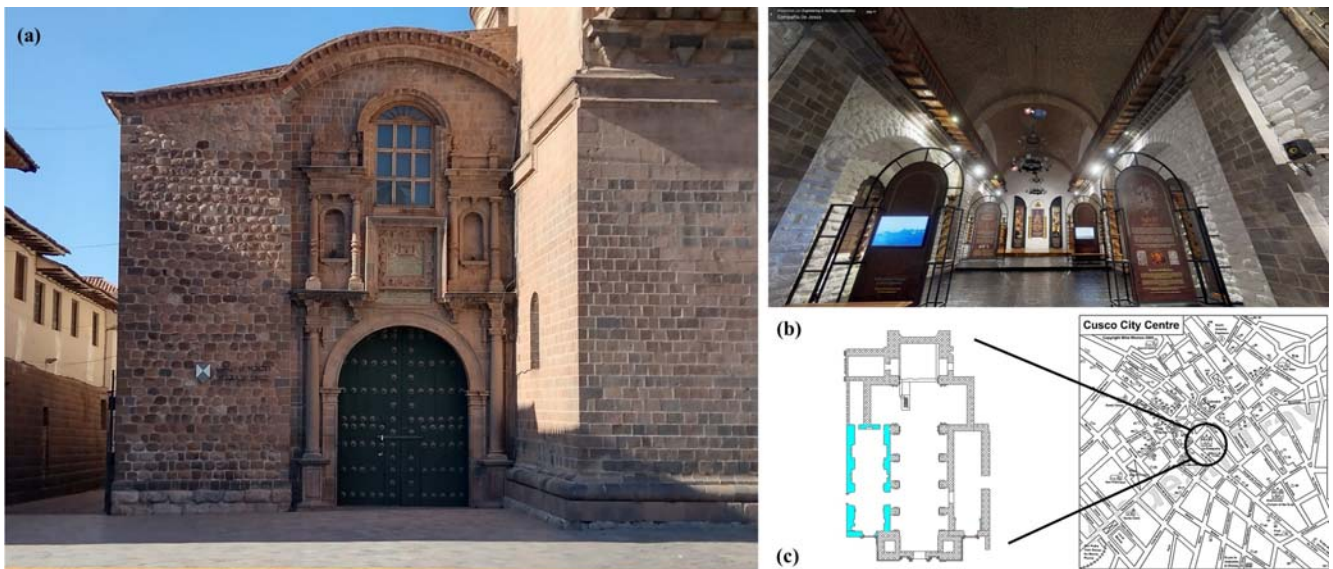
Fig. 2 Loreto chapel: (a) main façade, (b) interior, and (c) location
