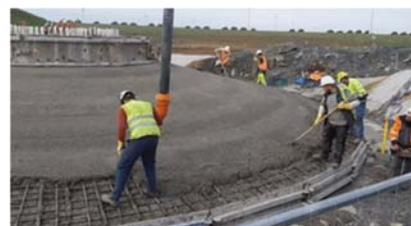
Fig. 4 Casting of a wind turbine foundation at Les Pierrots, France
