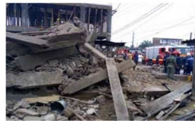
Fig. 1 Collapse of four-storeys building in the Ndogbat suburb
