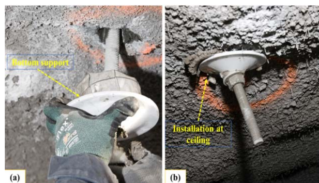
Fig. 15 Application of pucks on the tunnel ceiling a) during installation process, b) after installation of puck
