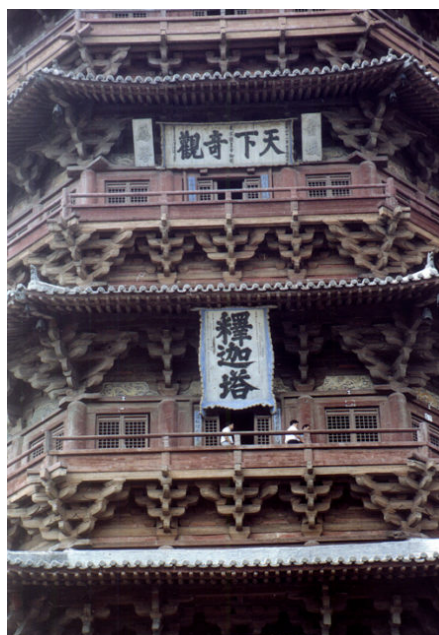
Fig. 2 Dougong bucket structures on the exterior façade of Sakyamuni Pagoda of Fogong Temple [22]
