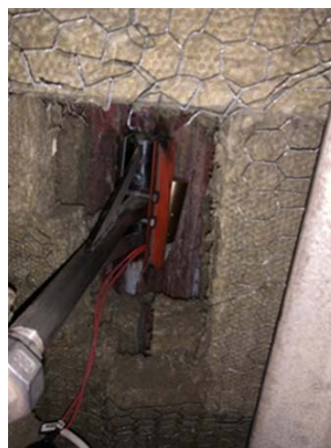
Fig. 5 Temperature sensor and heater installation
