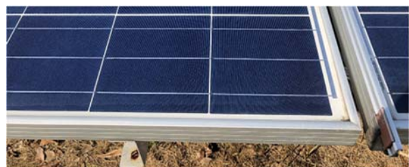
Fig. 4 The PV module after cleaning (PV module-1)
