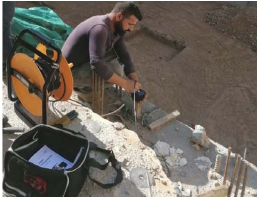
Fig. 6 Taking inclinometer readings at final excavation level
