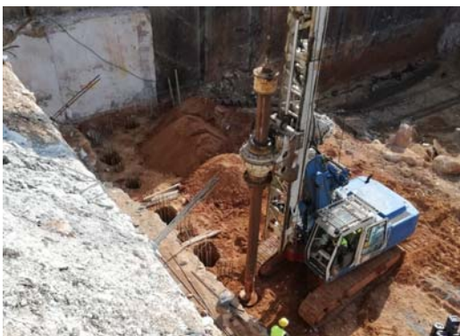
Fig. 3 Pile holes drilled to a depth of 15.0 m
