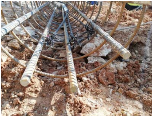
Fig. 2 Steel reinforcement structure
