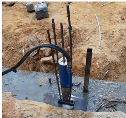
Fig. 5 Tensioning strands using a Mono jack
