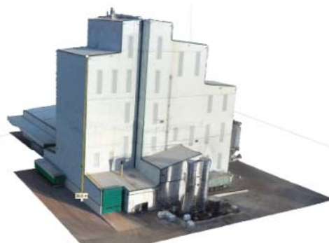
(b) Photogrammetry DTM, 30.60 m
