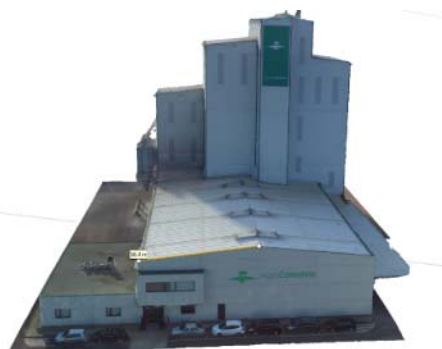
(b) Photogrammetry DTM, 16.4 m
