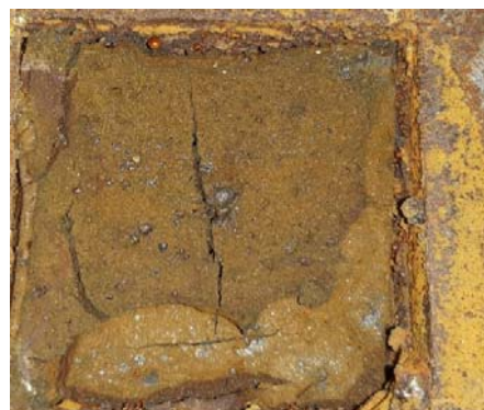
Fig. 7 Cracks observation at the surface of sample
