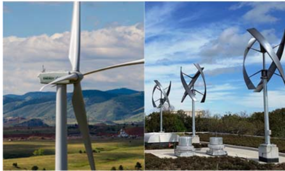
Fig. 12 Horizontal vs. Vertical Axis Wind Turbines
