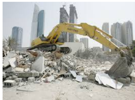
Fig. 3 Demolition of buildings [10]
