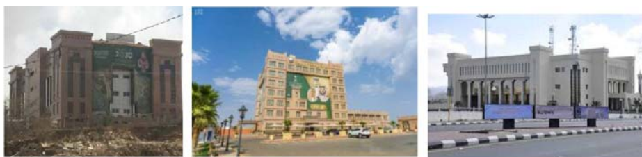
Fig. 4 Revival by imitation in projects Ministry of Transport building, the secretariat building and the Emarah building
