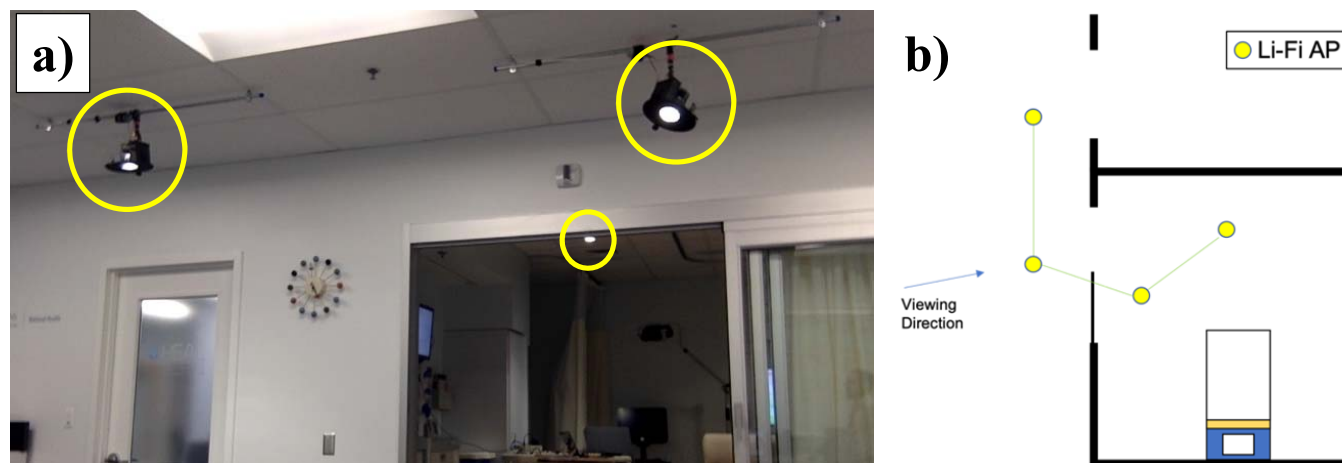
Fig. 1 Li-Fi Access Points in the Mock ICU (a) and a blue print of the location of the Li-Fi APs (b) showing the viewing angle of the picture
