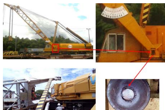
Fig. 1 The accident occurred with the railway crane due to the fall of the hoist by the fracture of the two support pins
