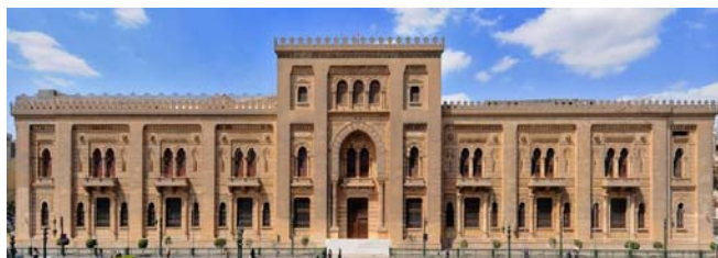
Fig. 8 The Museum of Islamic Art in Cairo was damaged by a bomb in 2014. It reopened in January of 2017. (Photo: Gérard Ducher, CC BY-SA 2.5)
