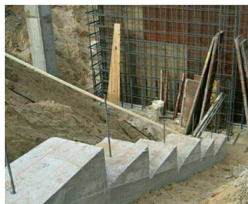
Fig. 1 Execution of stepped foundation in sloping lands
