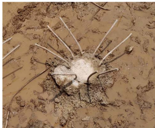
Fig. 2 Condition of prepared pile head
