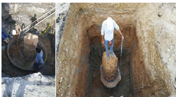
Fig. 2 Measuring the diameter and using the cement rings
