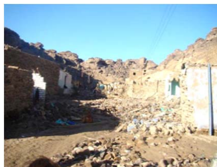
(b) Flood damaged urban areas
