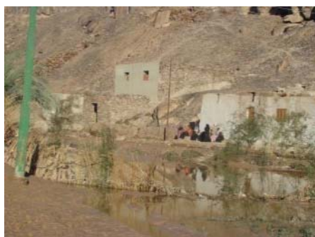
(b) Buildings destroyed by flood waters
