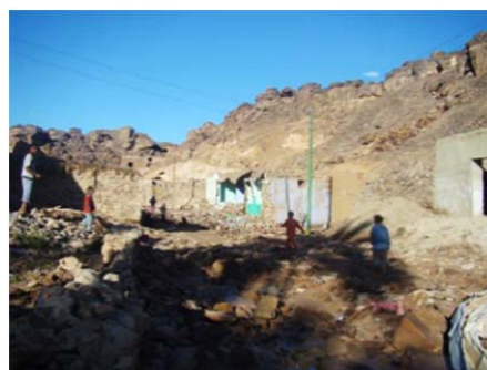
(a) Houses destroyed by deluge
