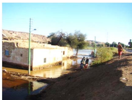
(a) Roads destroyed by flood waters
