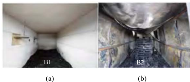
Fig. 10 (a) The interior of the fire simulation for Steel room, (b) The interior of the fire simulation for AAC wall systems after the fire
