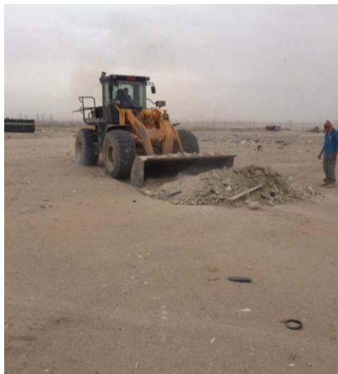
Fig. 1 Spade Tractor at the Site Reclaiming the Material
