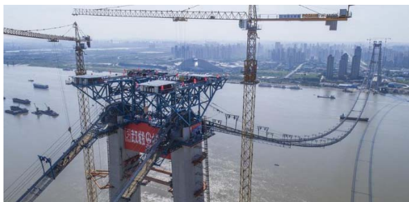
Fig. 8 Yangsigang Bridge (open source image)
