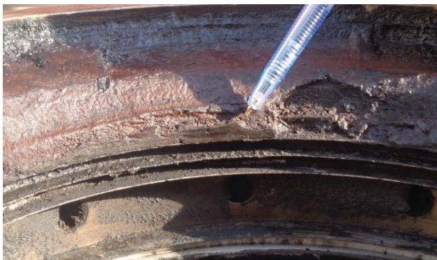
Fig. 13 Shedding of coke deposits after getting rubbed
