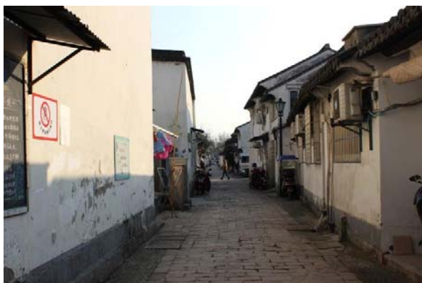
Fig. 5 Residential buildings of the Qinchuan Stream area
