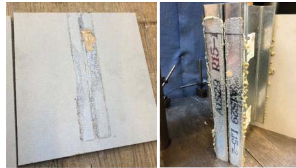
Fig. 4 Timber board and steel joist interface upon failure in specimens with adhesive only (P1.5-A)
