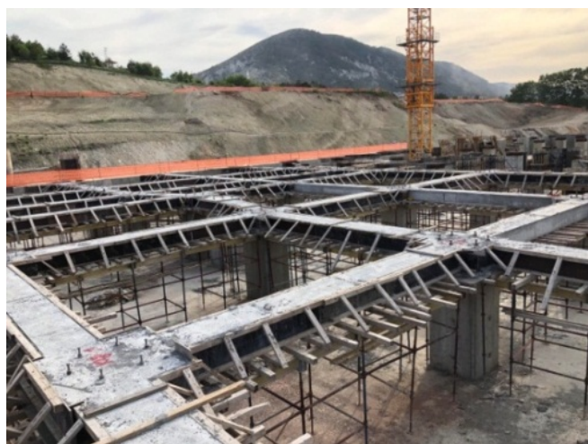
Fig. 3 Field application of the project
