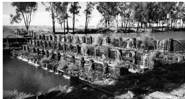
Fig. 1 Greenup timber crib weir [3]
