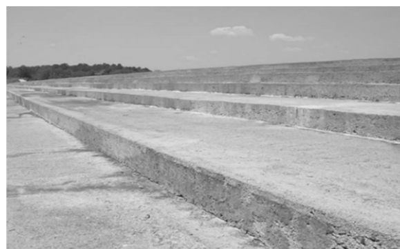
Fig. 7 RCC stepped spillway/overtopping protection of the Tholocco Lake dam [19]
