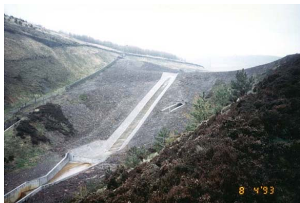
Fig. 5 Wedge concrete block spillway on the Brushes Clough dam [3]
