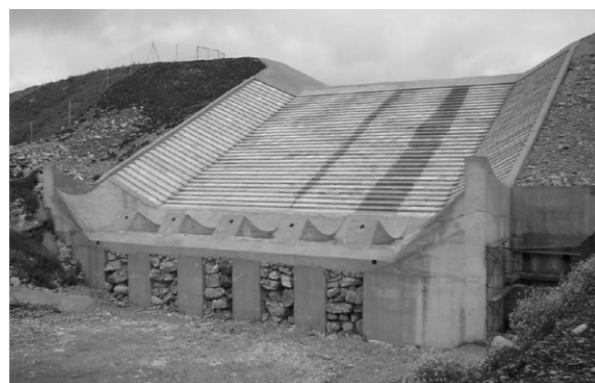
Fig. 6 Wedge-shape concrete block spillway of Barriga dam
