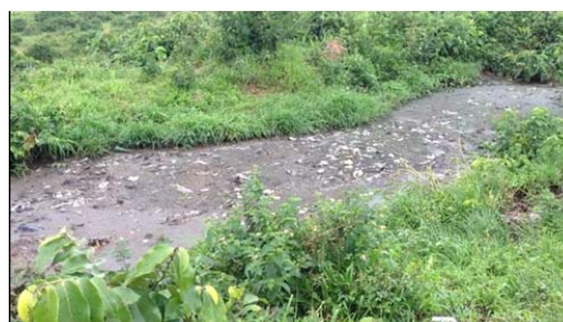
Fig. 3 (c) Trench for dewatering/separation of water from concentrated household sewage sludge
