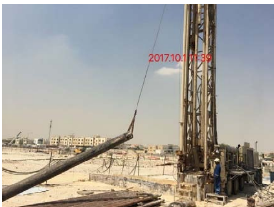
Fig. 12 Drilling rig for FPS 14, Site 8 (Al Dayeen) DM1A
