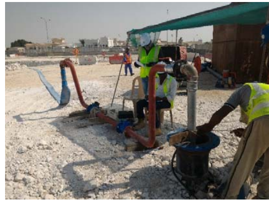
Fig. 21 Pumping Test Set-up
