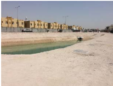
Fig. 20 General View of EFA Pond with Completed Manholes for Wellhead Assembly
