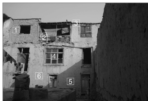
(b) A mixed type of house: 1 – Fired-brick wall, 2 – Wooden protected balcony, 3 – Mud roof, 4 – Wooden window, 5 – Mud–straw plaster, 6 – Adobe walls
