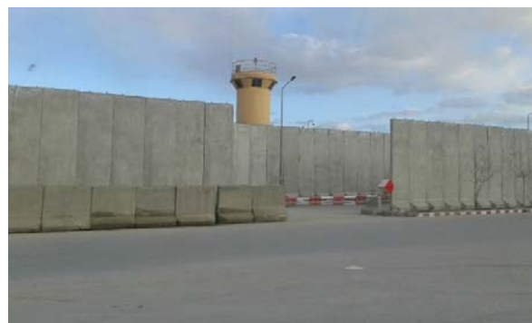
Fig. 1 T-Walls in front of one university in Kabul, (located on street and footpaths)
