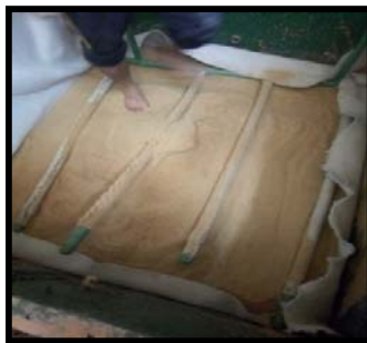
Fig. 3 Drainage system under clay layer
