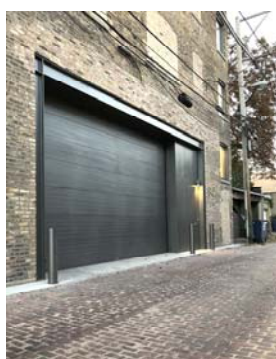
Fig. 10 South-facing loading dock door opens up to east-west alley
