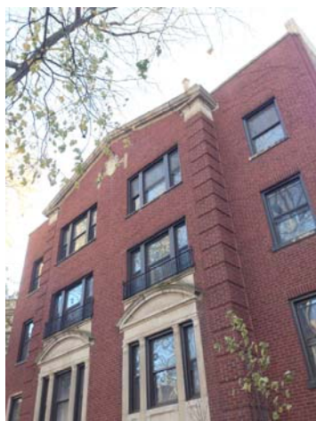
Fig. 7 Front faced of Wrightwood 659, pre-interior demolition
