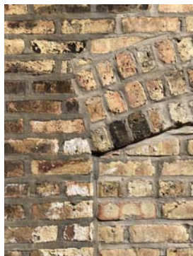
Fig. 14 Former window, now blind, south face of Wrightwood 659
