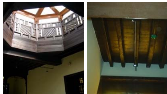
Fig. 10 Structure domes and wooden beams
