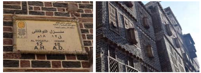
Fig. 23 Pictures of the façade of El Toktately House
