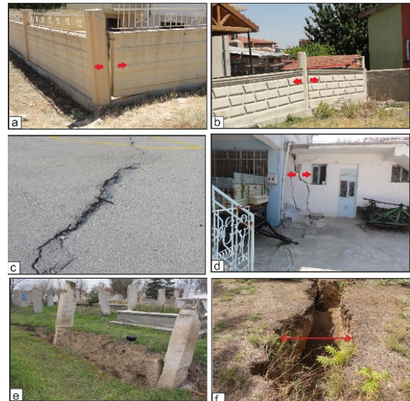
Fig. 3 The Surface deformations observed within the Bolvadin settlement area: (a),(b) The divergence of garden walls of some buildings located on the surface fault near the Park Akcan, (c) Linear deformations on asphalt pavement of the school garden, (d) Extensional cracks in some buildings located on the surface fault (e), (f) Deformations on graves
