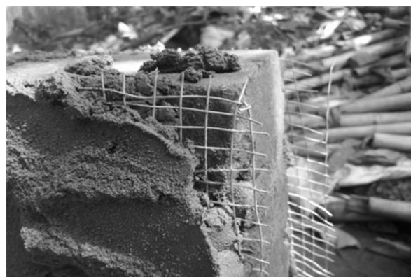
Fig. 4 Brick Wall After Applying of Ferrocement Coating
